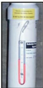
A liquid gauge, or manometer is used to verify that the system is operating properly
