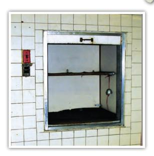
This is the dumbwaiter involved in the Schenectady, NY incident. There were no interlocks on the dumbwaiter. The doors were nailed in the open position. Workers were supposed to use a bell, which is not an appropriate communication control, to alert staff on the other floor before starting the dumbwaiter. In fact, the bell was broken.
